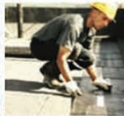
FLAT TOP ROOF
